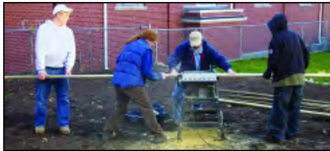
Ripping planks for the porch on 13 Steere Ave.
