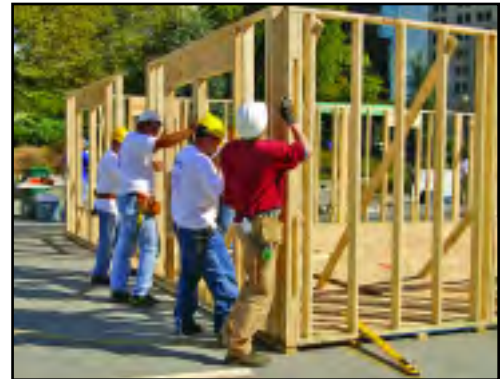
Walls were raised to test the "fit" prior to shipping to Mississippi. More pictures, Pg 4.
